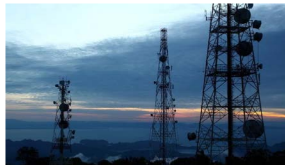
Dobson Tower Foundations, NEPA, & SHPO Provided designs and construction engineering services for over 130 cell towers located throughout the State of Alaska. 2001 to 2009.
