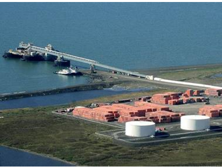
Red Dog Mine WWT Plant Provided the design, procurement and construction engineering services for the new WWT Plant. 2004 to 2005.
