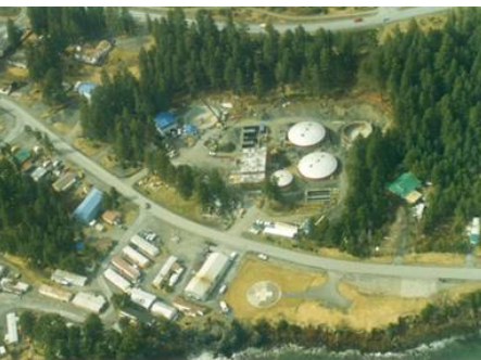
Kodiak Wastewater Treatment Plant Provided the design and construction engineering services for the new
