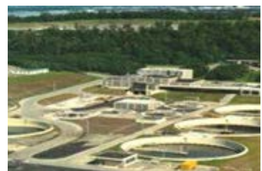
AWWU WWT Generator & Fuel Systems Provided the upgrade design for the AWWU WWT Plant standby generator and fueling system at seven separate sites. 2009 to 2011.
