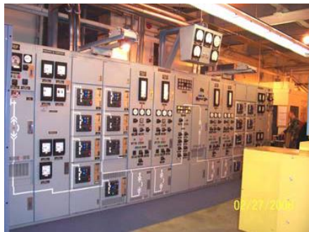
ALCOM Headquarters Renovations Provided the design support for the demolition of the existing facility and construction of the new headquarters buildings. 2007 to 2009.
