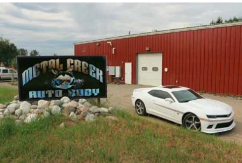
Metal Creek Auto Body Shop Provided the design and construction support for the new 8,000 square foot Metal Creek Auto Body Shop in Palmer, Alaska. 2005 to 2006.
