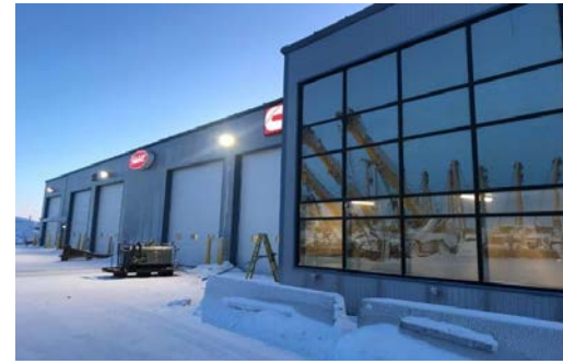
Price Gregory Maintenance Shop Provided the design and construction support for the new 20,000 square foot Price Gregory Light Duty Truck and Heavy Equipment Maintenance Shop in Deadhorse, Alaska. 2016 to 2017.
