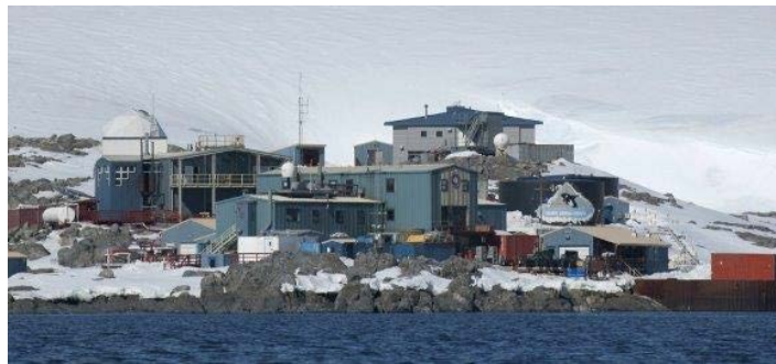
Palmer Station Pier Replacement Provided the design for a new pier and shore facility at Palmer Station on Anvers Island, Antarctica. 2015-2017.
